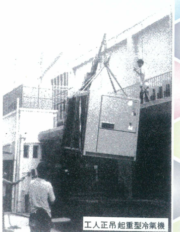
The installation of air conditioners in library and school hall
